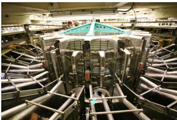
Center Section Installed
