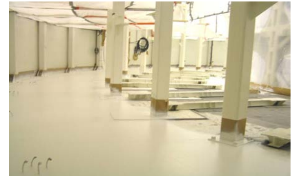
Tank Modifications Completed
